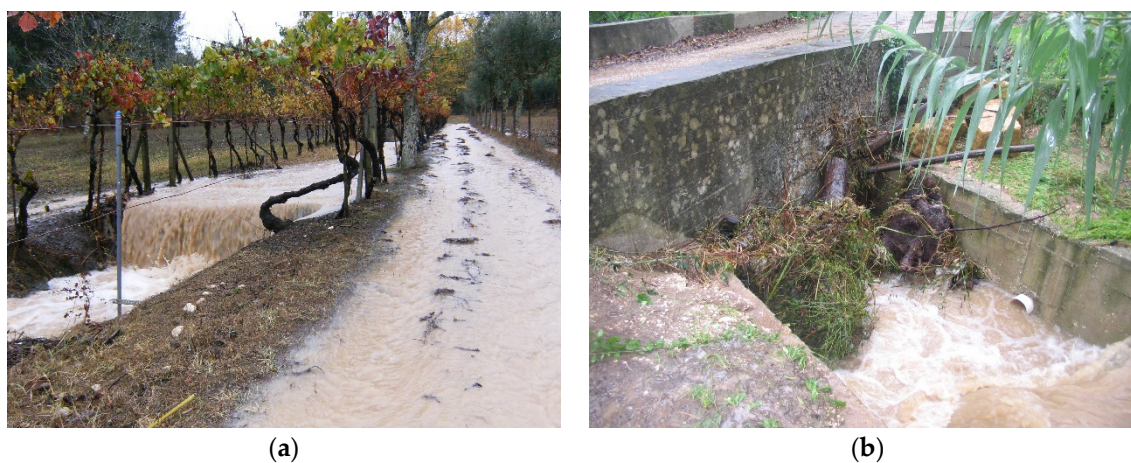
Figure 4. Causes of erroneous measurements of high peak discharge during major storm events, leading to lower observations at upstream gauging stations than in real conditions. (a) Stream overflow due to constructed channel section constriction in Quinta sub-catchment, to allow people and animals to cross the stream; and (b) partial blockade of hydraulic infrastructure in Covões sub-catchment with sediment and litter carried during high-intensity storms.
