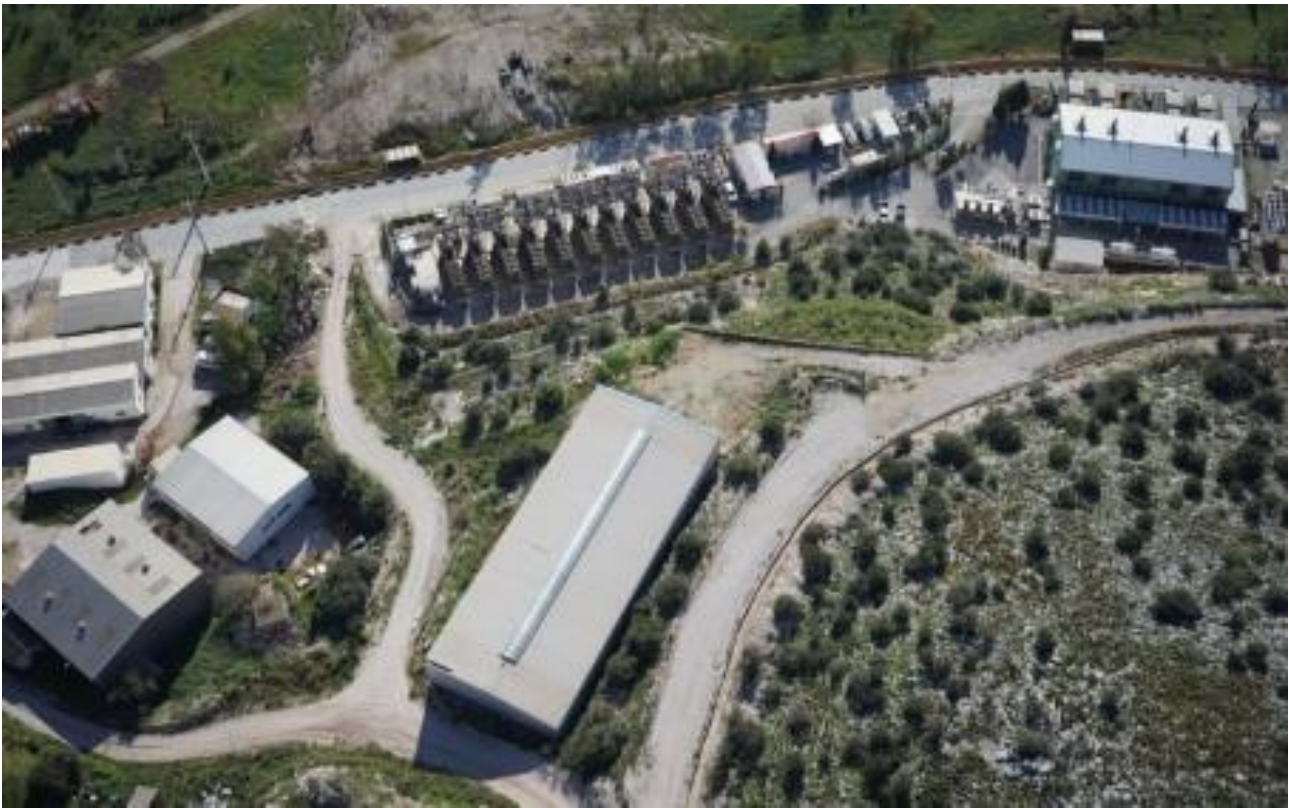
Figure 2: Overview of the Ano Liosia Landfill Biogas Power Plant
