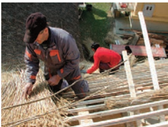
Figure 5: Making straw roof, Sovjak, Slovenia
