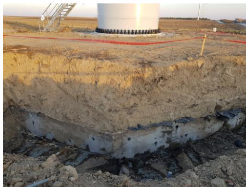
Figure 1 – Concrete elements (foundations) of wind tower
