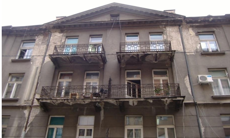
Figure 1. Front view of the main front façade of the object
